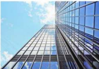
2 Sided Structural Glazing - 2 SSG
