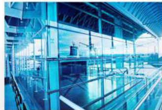
4 Sided Structural Glazing - 4 SSG
